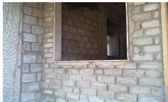
Fig. 2 Fly ash brick Masonry at Palghar.
