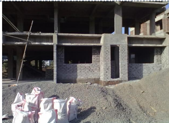
Fig. 3 Fly ash brick Masonry at Boisar.
